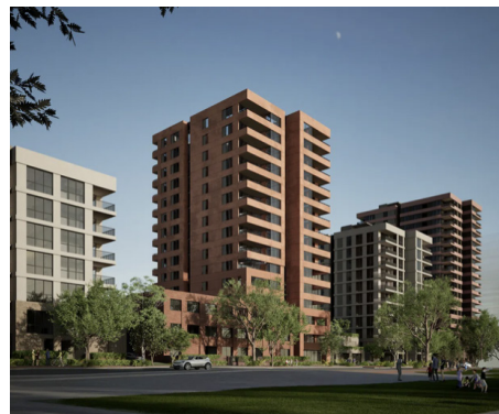
Court Place, Subiaco, social and affordable housing project (Image source: CHL)
